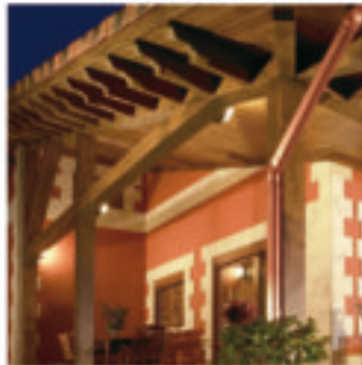
Porches with eaves covered with wood and beams in laminated wood
