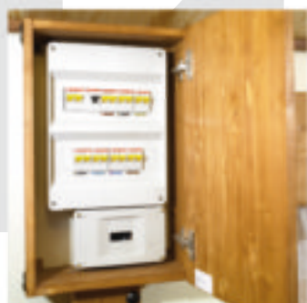
Fuse box protected by a differential magnetothermal switch. Electric Installations According to the regulation for low voltage (RD 842/2002)
